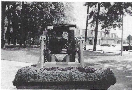
Placement of crushed stone with bobcat.
