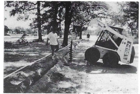
Bobcat used to drill holes for bollards
