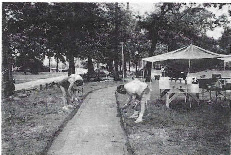
Putting finishing touches on the completed walkway.
