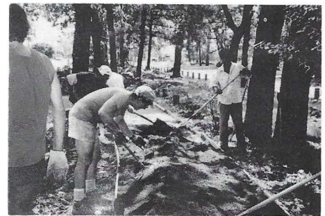
Crushed stone being spread on walkway.
