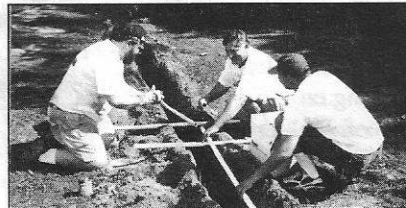
Installing the irrigation system, Fall 1998
